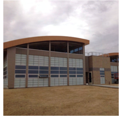
NASA Facilities Support Center , Edwards Air Force Base, CA | LEED Platinum, NC
