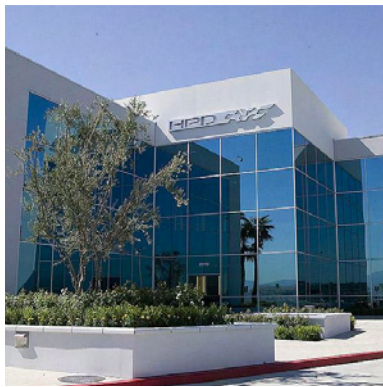
Honda Performance Development Facility , Valencia, CA | LEED Silver, O+M: Existing Buildings
